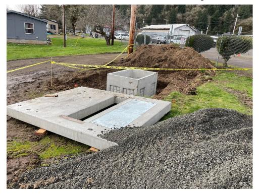
The new transformer vault has been set and is awaiting backfill.
