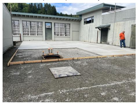
Underground conduit are installed for the Panel Room, the new retaining wall has been formed, and the vapor barrier for the Panel Room slab is being installed.
