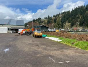
The building pad has been excavated and base rock installed.
