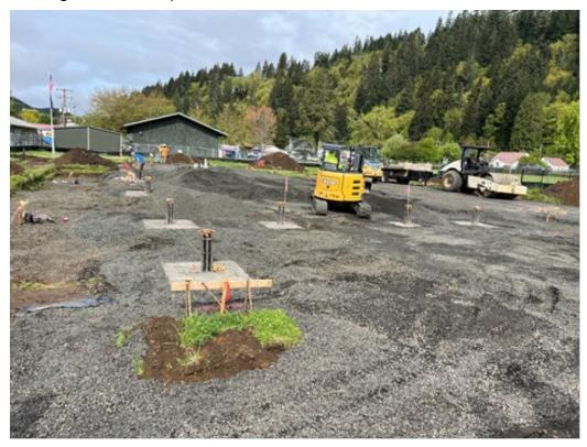
Compaction and grading for the building slab is in progress.
