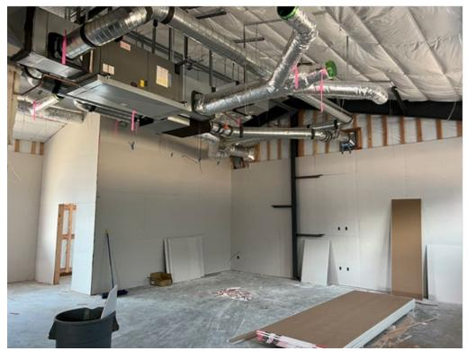
HVAC duct installation is being completed and lights have been installed in the shop.
