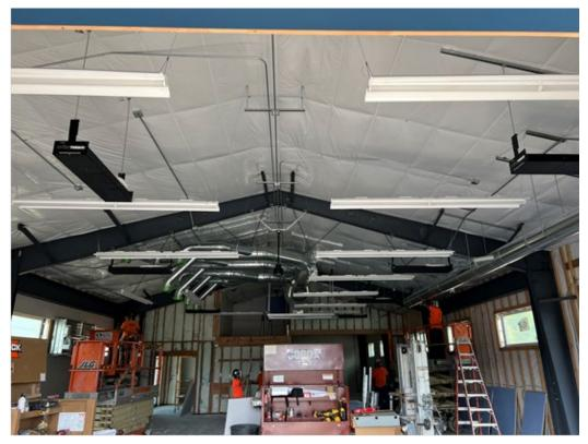
Electrical, plumbing, fire alarm and data rough-in are complete.
